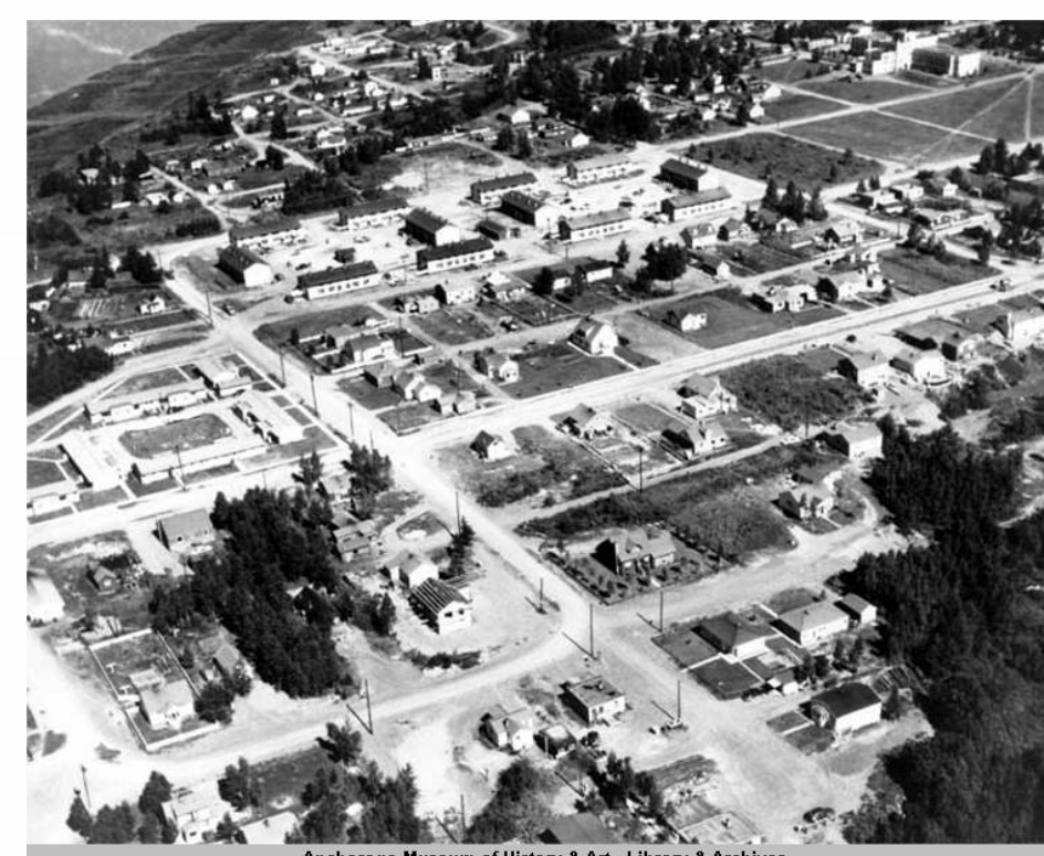
VIEW OF ANCHORAGE SOUTH OF 9TH AVENUE CIRCA 1940s, FROM THE ALASKA DIGITAL ARCHIVES
