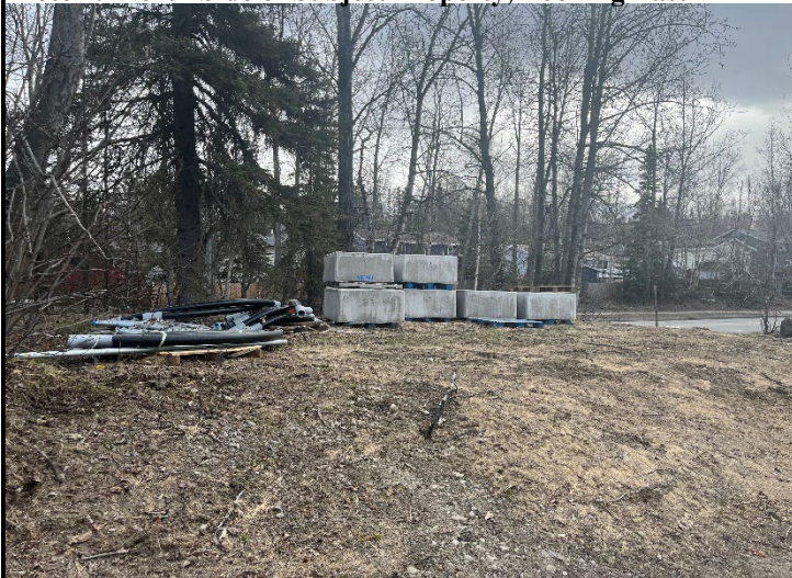
Photo 3. Pipes and Concrete Blocks, Looking East
