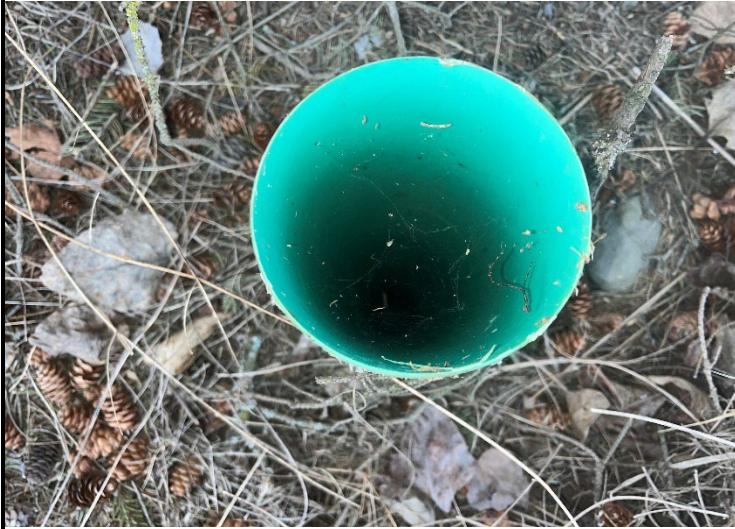
Photo 9. Possible Septic Vent Pipe
