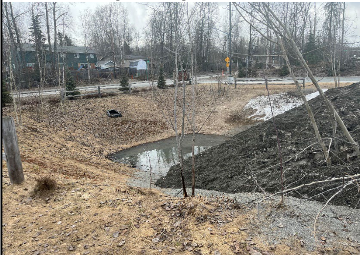
Photo 11. Drainage Pipe and Apparent Settling Pond, Looking SE
